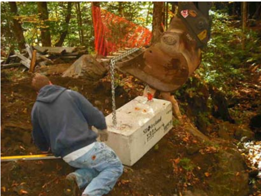
Paul Torrey installing the precast concrete blocks
