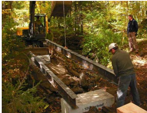
Matt Z installing the 10" steel I-beams
